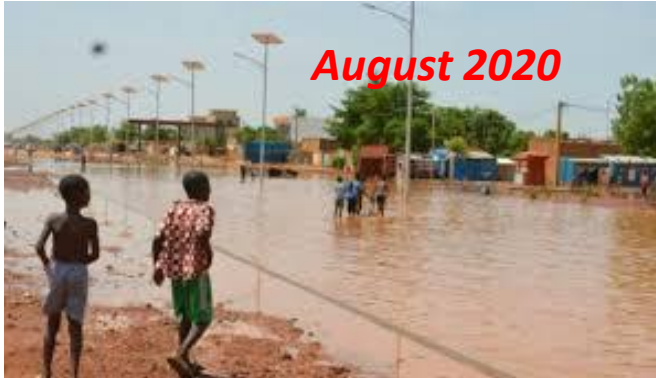
Fig 6: Main road flooded
