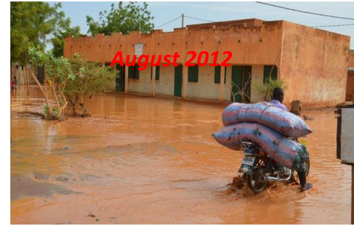
Fig 4 : School compound flooded
